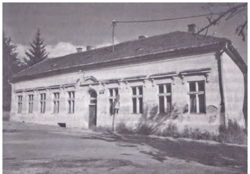
In 1992, the building of the former Jewish school in Lendava was pulled down. It was the only preserved Jewish school on Slovenian soil (source: Mirjana Gašpar, Beata Lazar, Židje v Lendavi , 1997).
