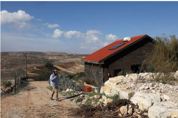
Esh Kodesh, an outpost near the Jewish settlement of Shilo in the West Bank
