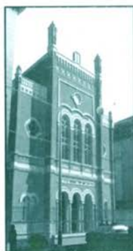
The Zagreb synagogue (destroyed 1941)
