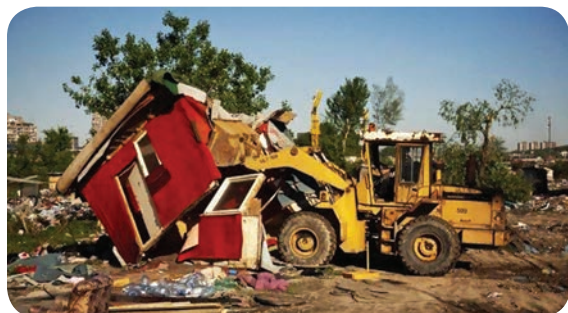
Forced eviction and demolition of the informal Roma settlement "Belvil" in Belgrade, in April 2012
