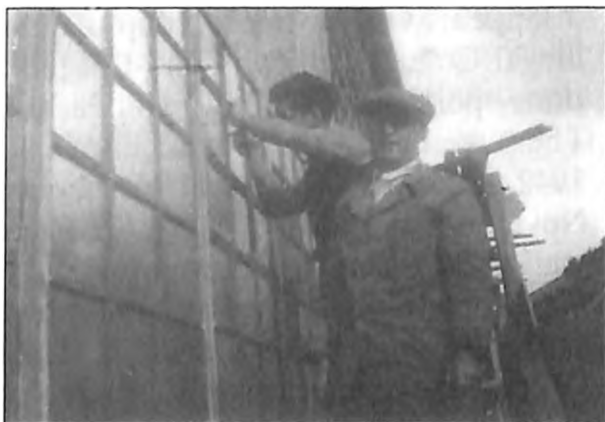
Dorde with his father, fitting windows in the factory building
